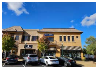
4357 TOWN CENTER BLVD, ST 220 EL DORADO HILLS
