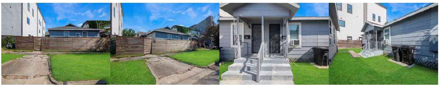
Front unit of the Fourplex Front unit of the Fourplex Back units of the fourplex Back units of the fourplex
